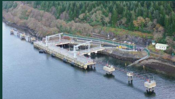
The Northern Ammunition Jetty at Glen Mallan following the completion of work. [Copyright VolkerStevin 2021]
