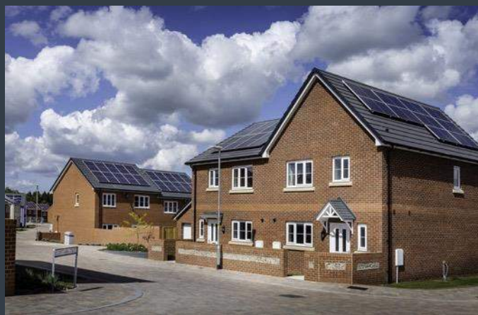
New housing at Larkhill, built under the Army Basing Programme.
