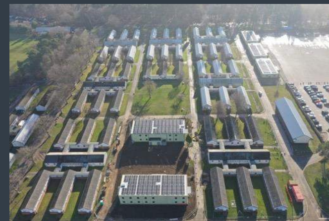
The latest double-storey NetCAP accommodation buildings allow for 104 bed spaces each and feature rainwater harvesting technology [Copyright: Reds10 Ltd]
